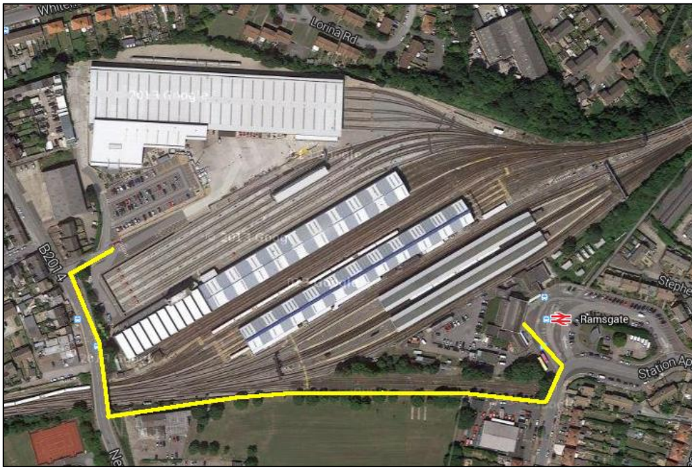
Figure 4: Route of 7- 10 minute walk between the Ramsgate Railway Station and Ramsgate Maintenance Depot (Source: Google Maps)
