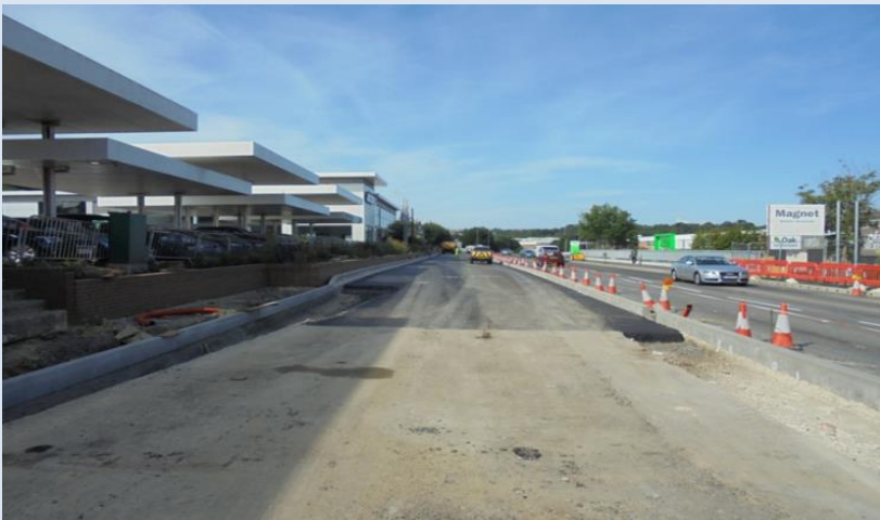
Retaining wall, high level kerbs and central reserve at BMW
