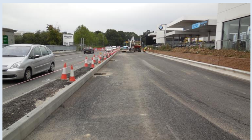
Retaining wall, high level kerbs and central reserve at BMW
