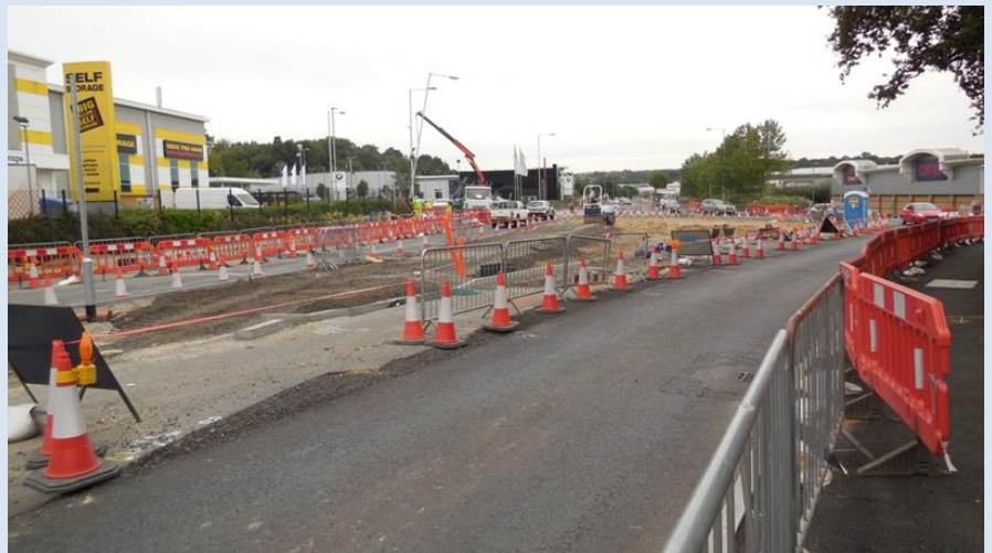
Construction of new gyratory at Great Lodge
