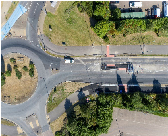
Aerial shot of completed phase 1 and 2 works
