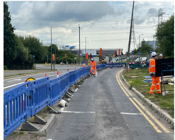
TM being set up for next phase of working
