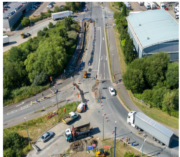
Rennie Drive junction aerial shot (north).
