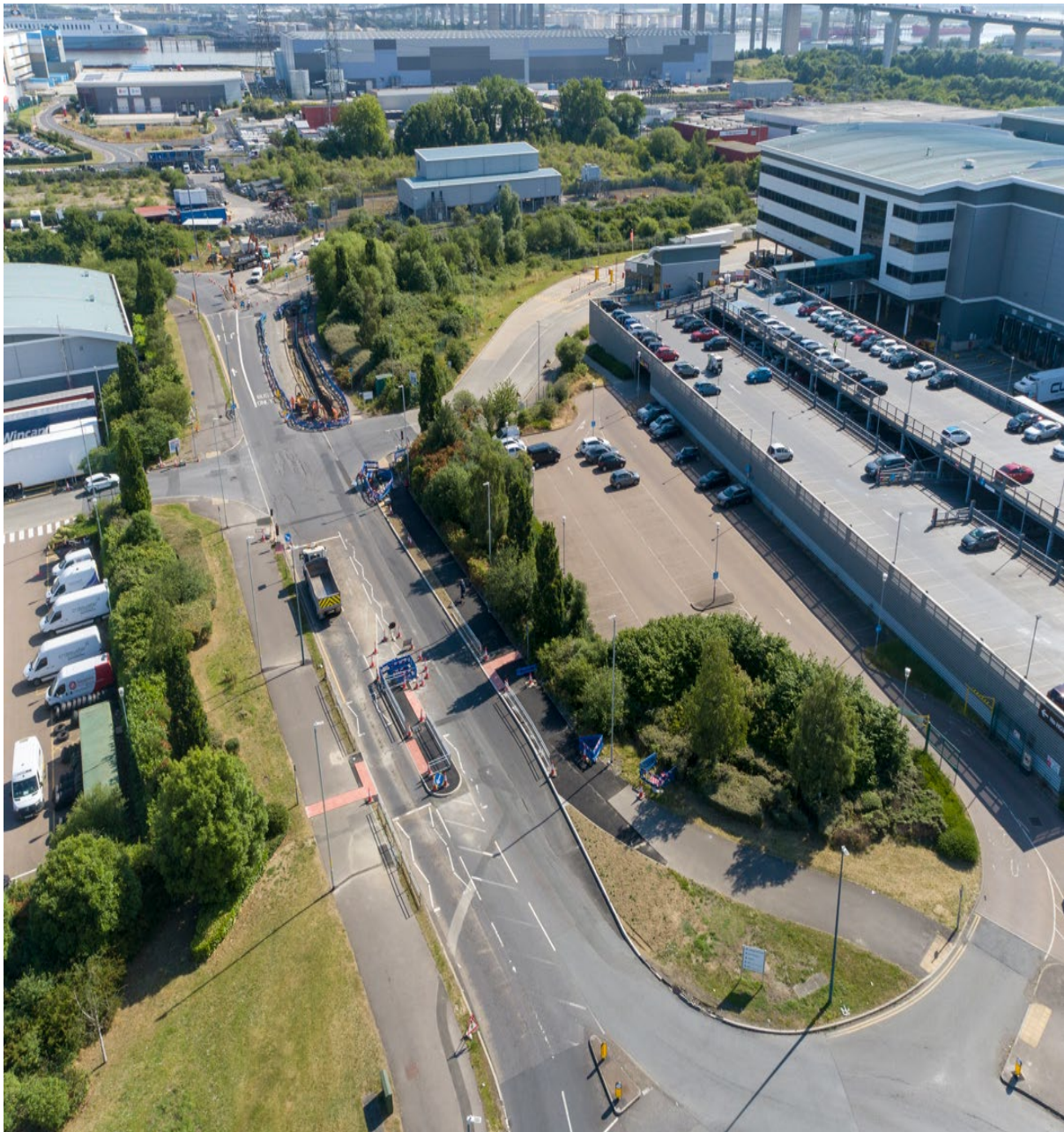
Aerial shot of the Rennie Drive Junction to show progress as of June 2024
