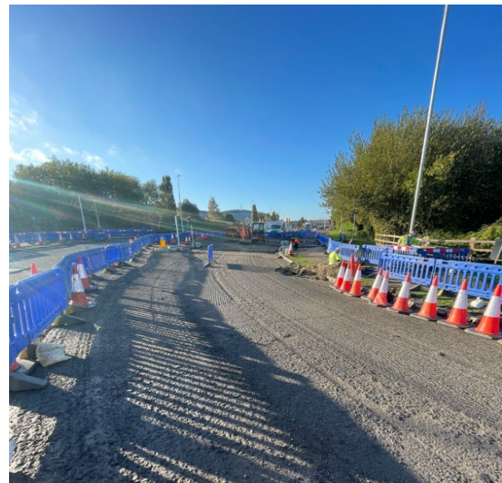
Carriageway milling within phase 6.
