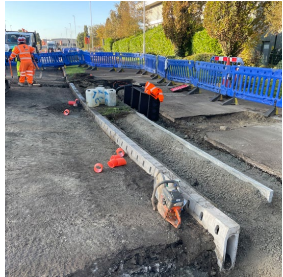
New Aco-Kerb drains that have been . Installed within phase 6.
