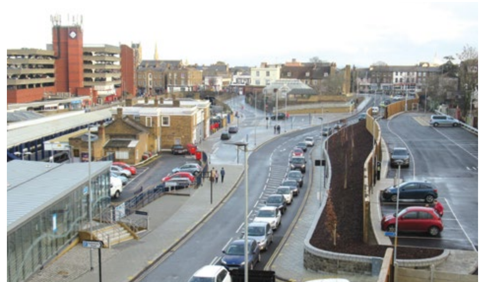
Rathmore Road completed improvements in Gravesend
