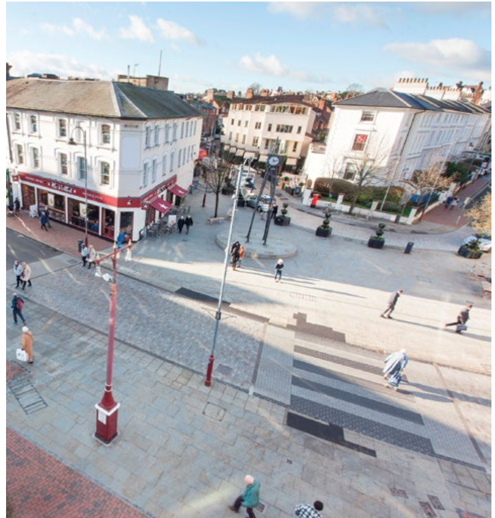
Public realm improvements at Fiveways, Tunbridge Wells
