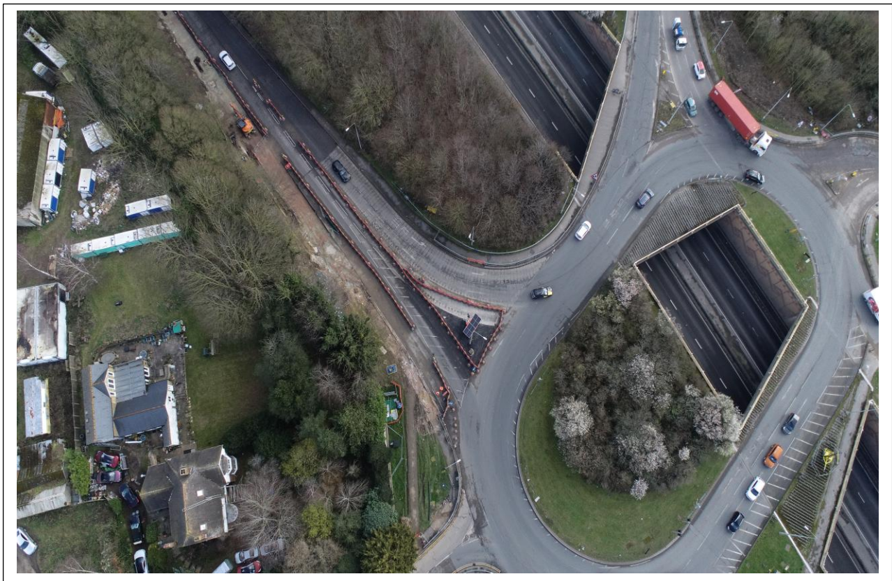
Aerial view of highway realignment works on Sheppey Way.
