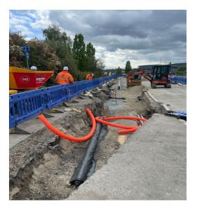
New traffic signals ducts being installed.
