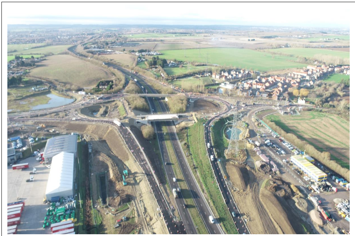
Works in progress
