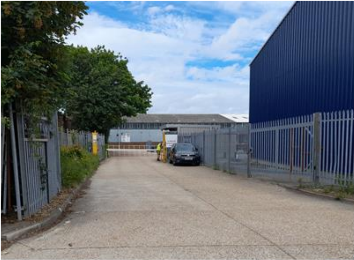
Figure 2: Haulage Entrance & Security Hut
