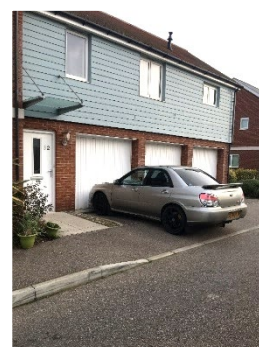
An example of poor design, resulting in footway obstruction due to an overhanging parked vehicle.
