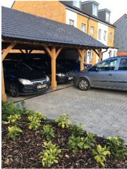
Tandem parking, with a car port space equating to 50% of the parking provision.
