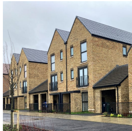
Car ports located to the side of buildings – Alkerden, Ebbsfleet.
